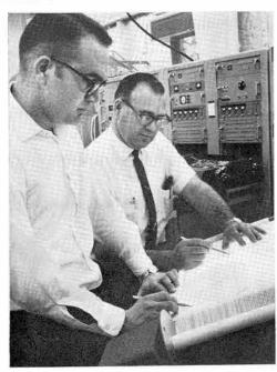
DATA SHEETS from QEST (Quality Evaluation Systems Tester) are checked by Harry Morris, left, and John Thomas. The computer-like QEST programs a sample weapon through complete parameters of performance. It must meet rigid standards. After systems check, weapon components are also checked for performance.
